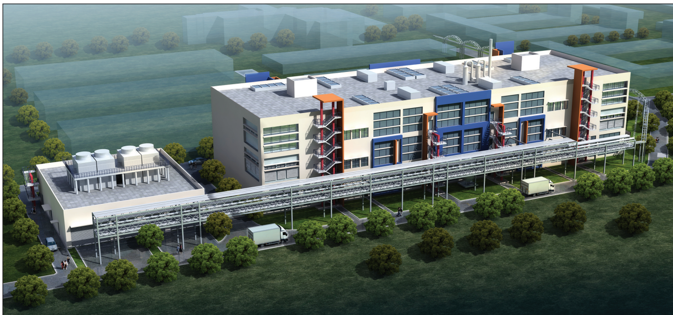
Figure 3. The new production plant and its utility building.
