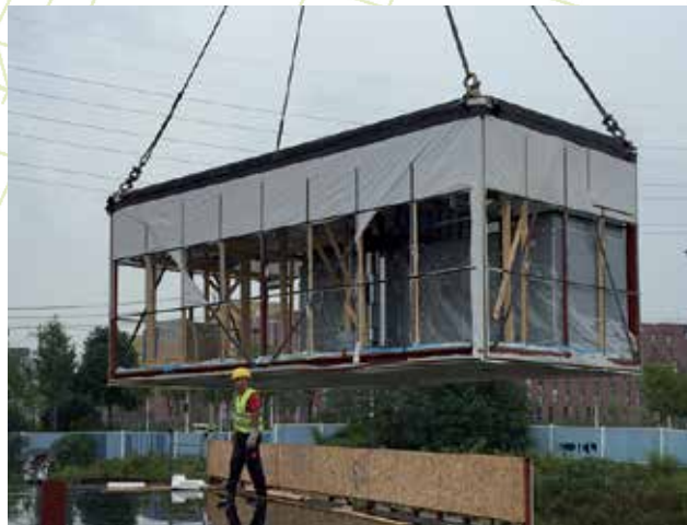
A crane places one of the 62 KUBio modular components that will become the GE Healthcare Life Sciences facility in Wuhan, China.
