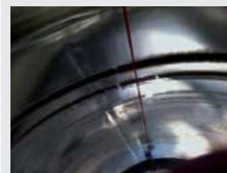
Figure 6 Visible rings in tank.
