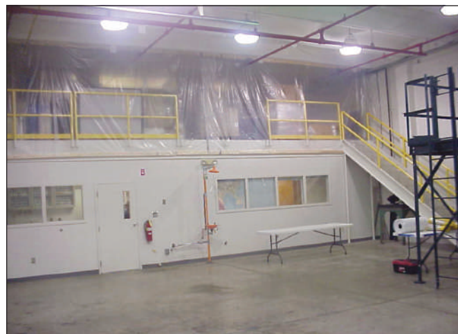
Figure 2. Mezzanine adjacent to test room, sealed off with poly sheeting with dust collector platform visible at the right.
