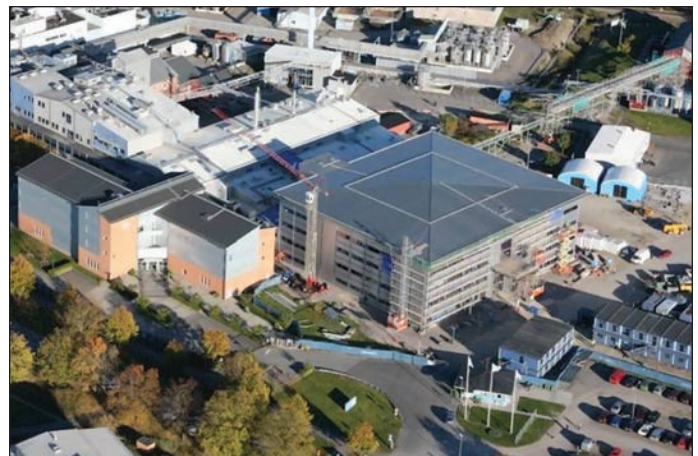
Bio 7 under construction.
