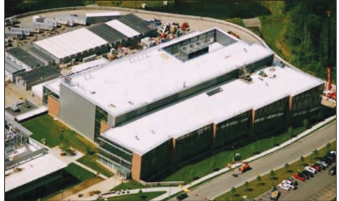
Aerial view of Project Atlas with trailers.
