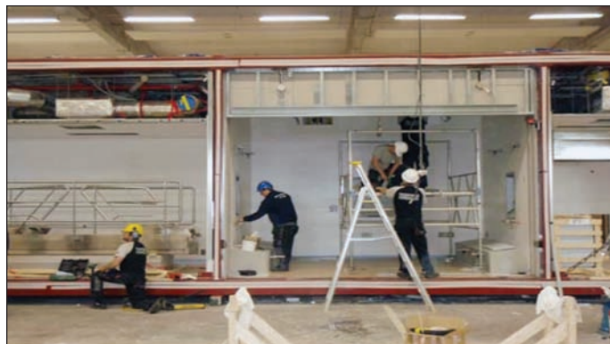
Module fit-out in Sweden.
