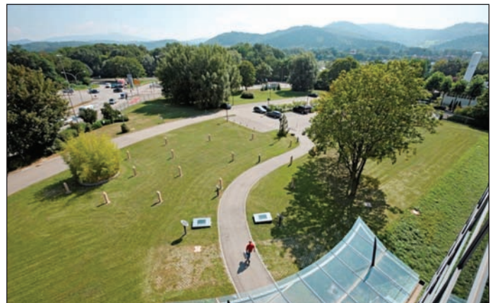
Energy tubes area in geothermal field.
