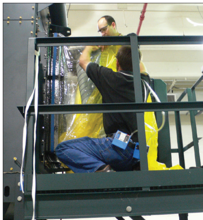
Figure 7. Operators performing BIBO filter cartridge change.
