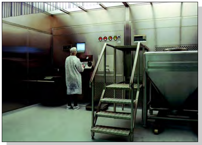
Figure 6. Typical downflow containment booth.
