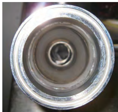
Figure 1. Residue deposits on recirculation pipe for granulate after CIP.
